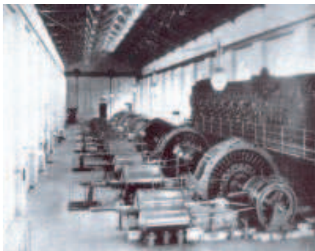
Figure 1: Steam driven electricity generators in Budapest (1895). Designed and produced by Ganz company (courtesy Elektrotechnika – Hungary)
