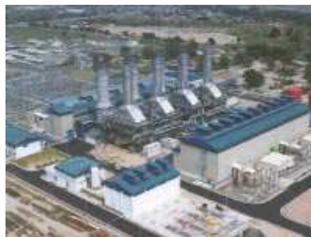
Figure 2: Combined-cycle power plant in Malaysia 2 \times 400\text{MW} (© Siemens)
